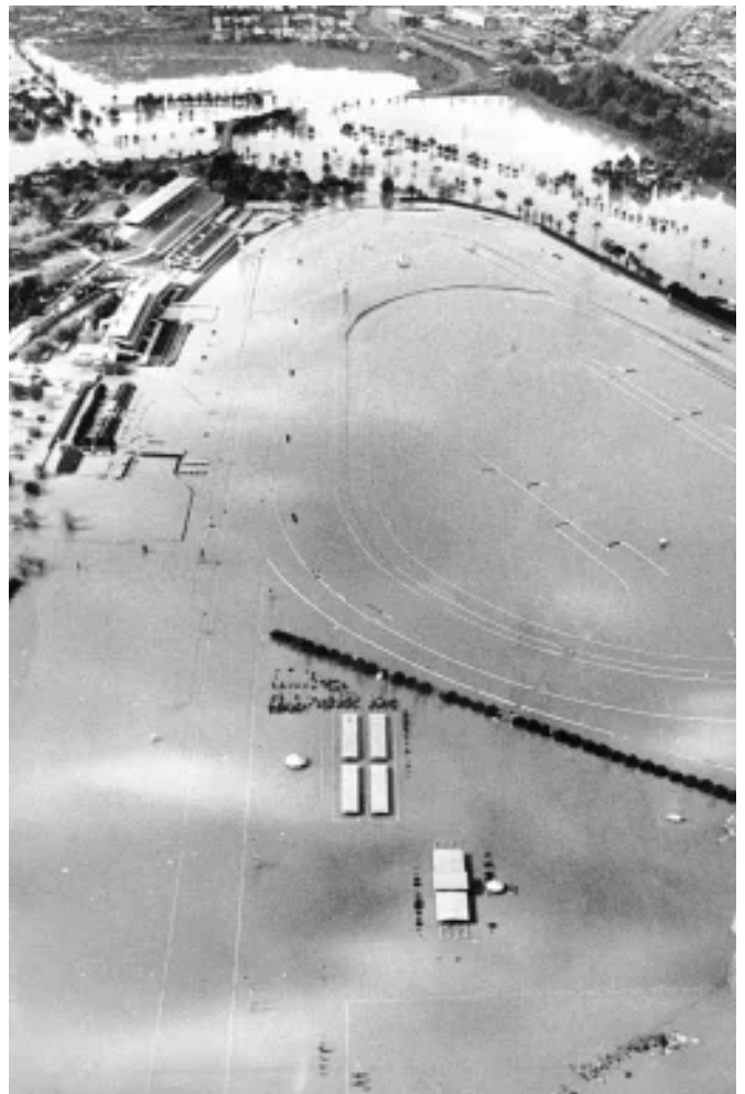
Flemington Racecourse submerged by the floodwaters. THE AGE ARCHIVES
