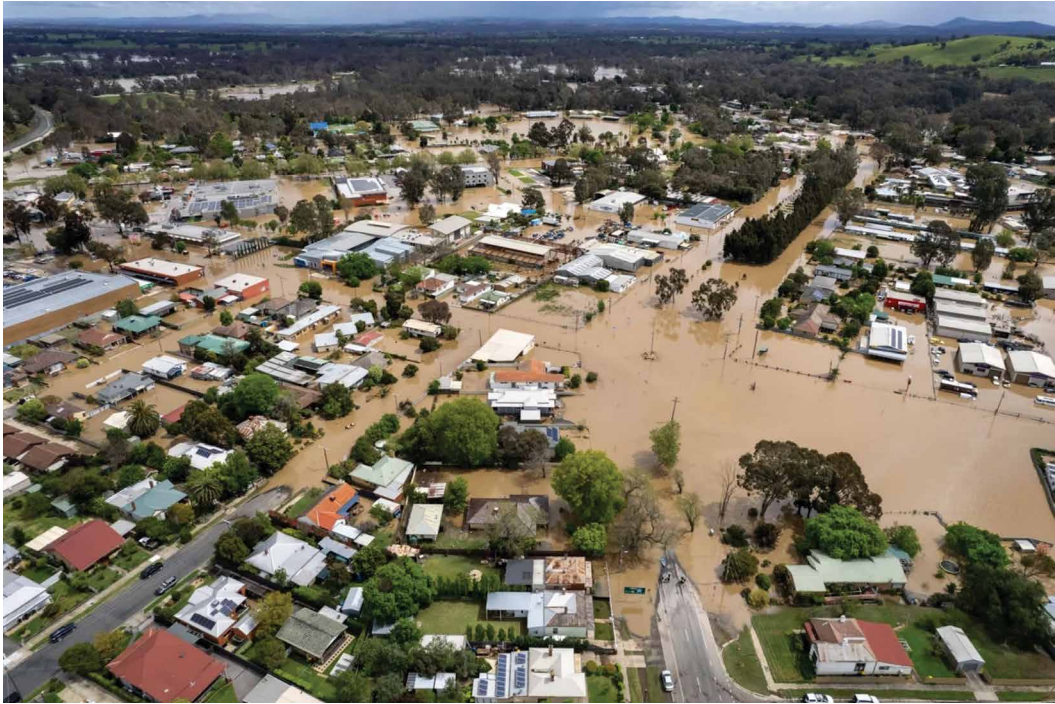
Figure 3.5 An aerial view of the flooding at Seymour in October 2022
