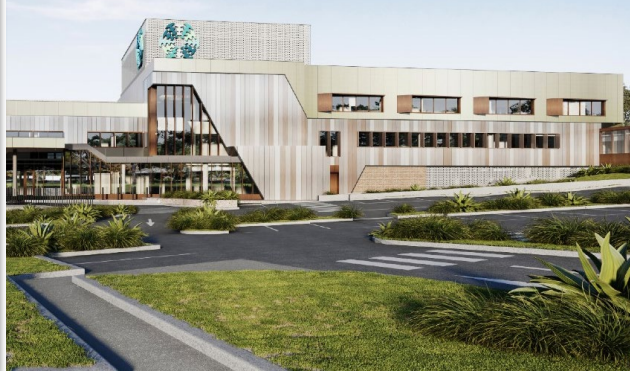
Wonthaggi Hospital expansion complete (Stage 1)
