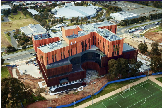
The Victorian Heart Hospital complete
