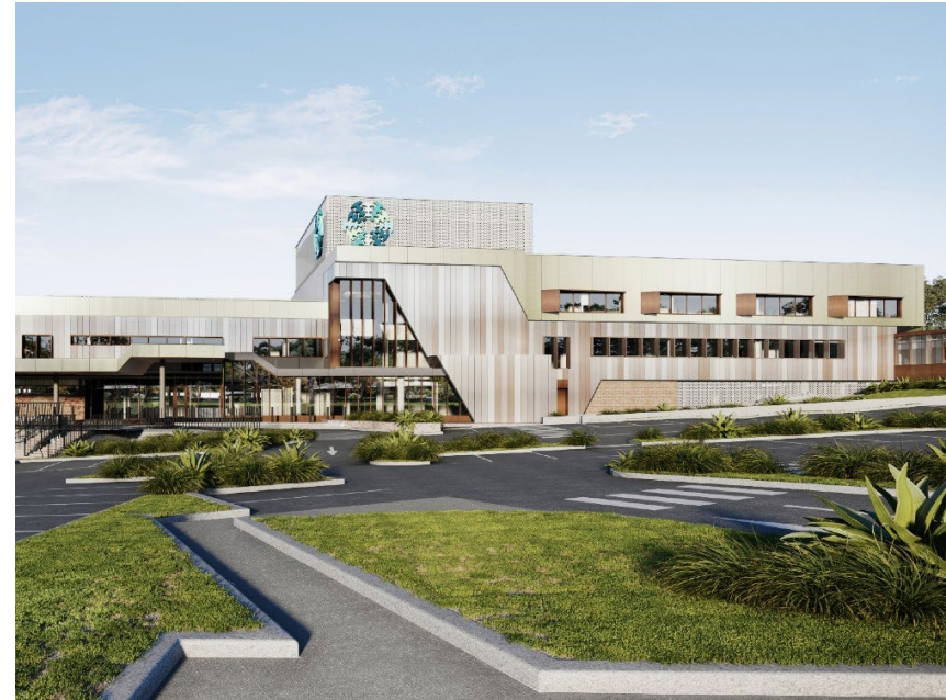
Wonthaggi Hospital Redevelopment
