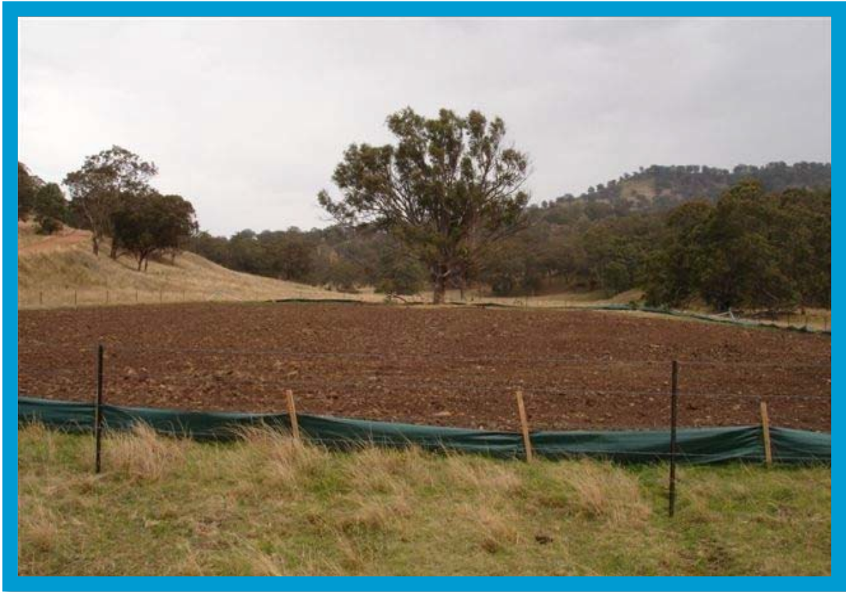
Figure 15: The same site during rehabilitation
