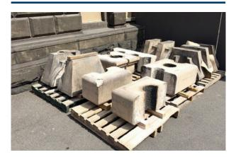
The entire chimney on the east facade was dismantled and re-laid as it was found to be leaning outward and structurally unstable.
