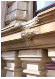
The refreshment wing balconies show a significant level of deterioration. Severe spalling of top rails is evident where pieces of previous repairs and existing stone have fallen away.
