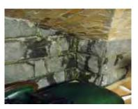
Water has penetrated the space below the front steps of Parliament House, causing extensive damage to the building interior, including Members' accommodation and storage areas.
