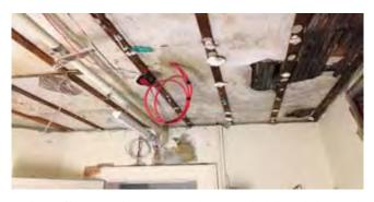
Evidence of historic and ongoing water damage to the lathe and plaster ceilings of spaces converted to Members' offices in 2011-12. These had been sheeted over with horse hair plasterboard.
