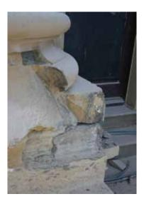
Above and below: Cracks, crumbling and deterioration to existing stone and previous repairs in library wing columns led to this stone falling away during restoration works.
