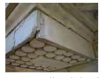
Stone restoration addresses the decay of features such as mutules and soffit carvings. The underside of these is deteriorating to the extent that a number of elements have fallen off when examined.
