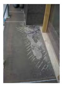
The bluestone blocks of the south wall ledge of Queen's Hall are delaminating. Water pools here and can penetrate the stone over prolonged periods, making the condition worse.
