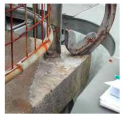
The original balustrades located on outside ledges of Queen's Hall highlight the potential problems of oxidised fixings spalling the existing bluestone stone structure. At all fixing locations of the balustrade the stone is severely cracked and large portions of the stone are missing at some fixing points.
