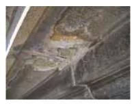
The cornice joints above Queen's Hall have deteriorated and pointing has failed. This allows moisture in to the underside of the cornice.
