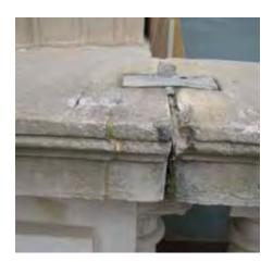
Balcony joints display signs of weakening through cracks and deterioration which is evident around existing dovetail connections. The integrity of the stone at these fixing locations is compromised and the balustrade structurally unsound.
