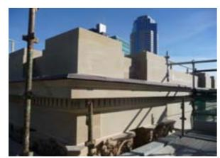
New stone and replacement copper flashing
